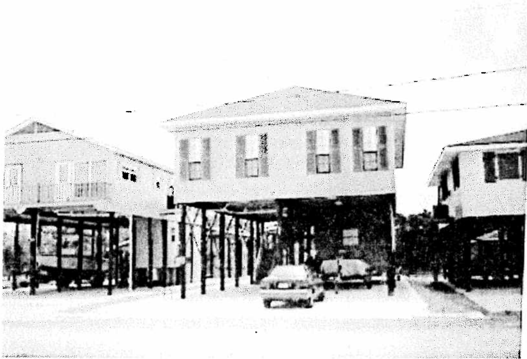
Figure I-7: Structure Elevated on Piles
