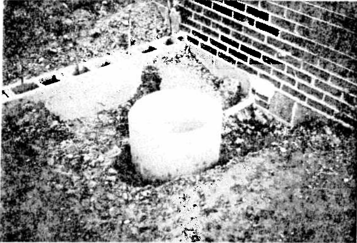
Figure VI-F24: Typical Patio Sump Pump Installation
