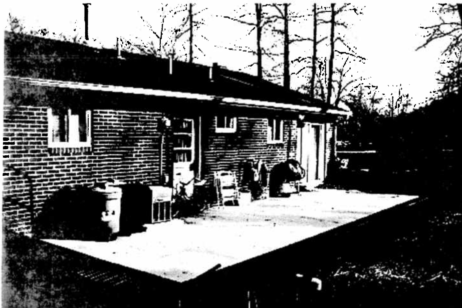
Figure VII-5.10: Sump Pump Outlet and Raised Air Conditioner Unit
