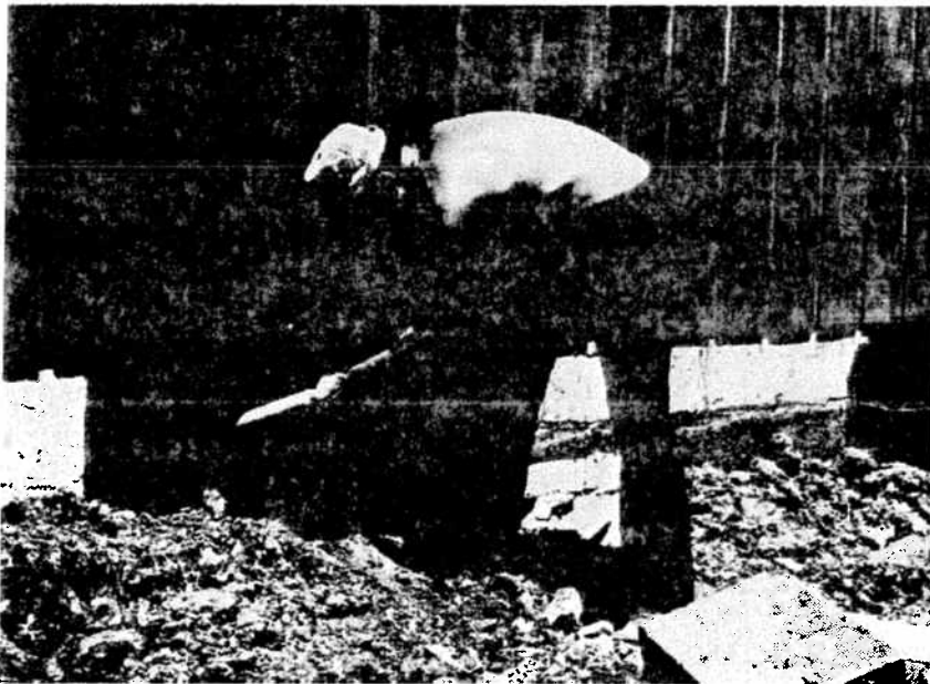
Figure VI-R5: Clearing Pathways Beneath the Structure for Lifting Supports
