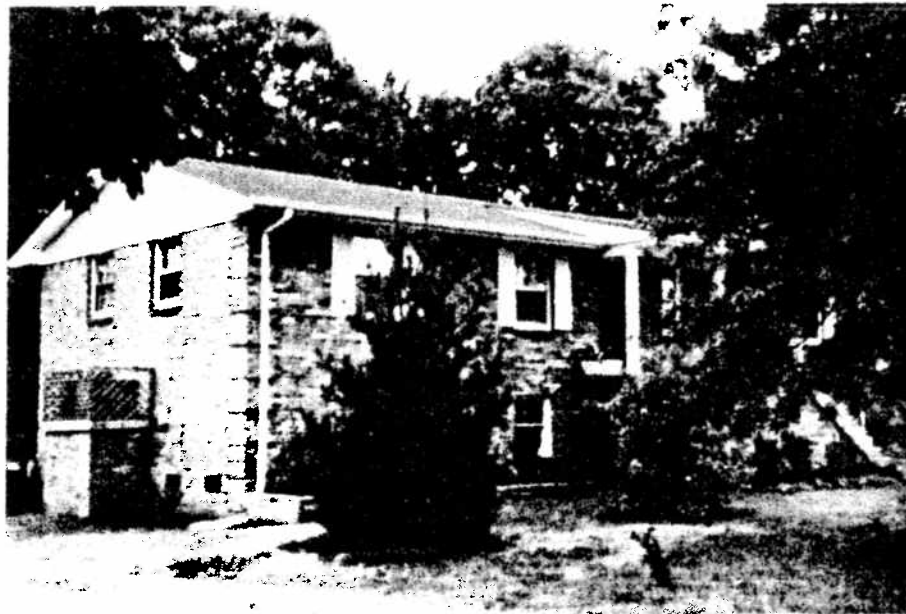
Figure VII-2.7: Example of a Home Raised With Air Conditioner Compressor Unit on Elevated Platform
