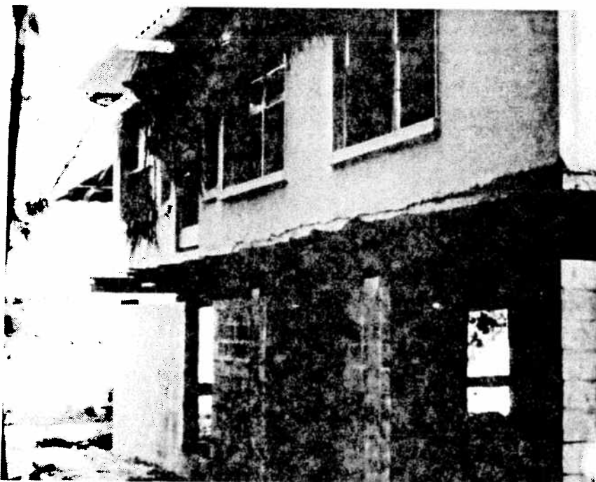
Figure VII-3.21: Breakaway Exterior Walls
