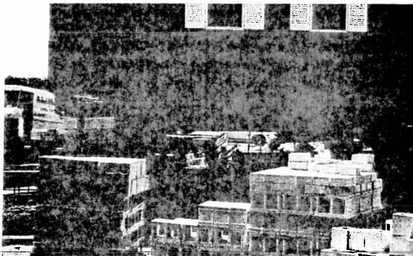
Figure VI-R18: Materials for New Foundation are Readied
