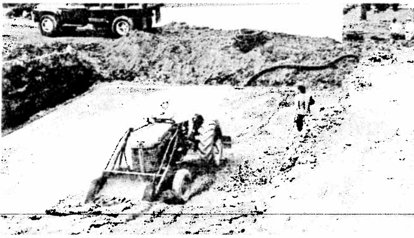
Figure VI-R16: Foundation Preparation at New Site
