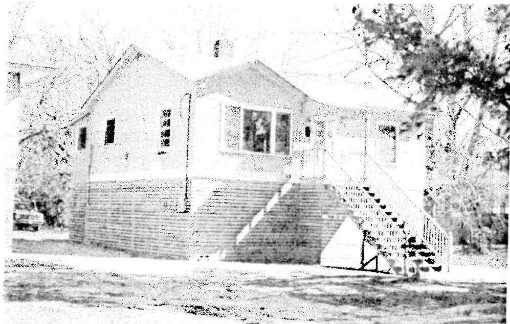
Figure I-5: Structure Elevated on Posts
