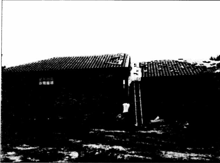
Figure VII-3.24: One Section of the House Has Been Raised, Prior to Insertion of Dollies
