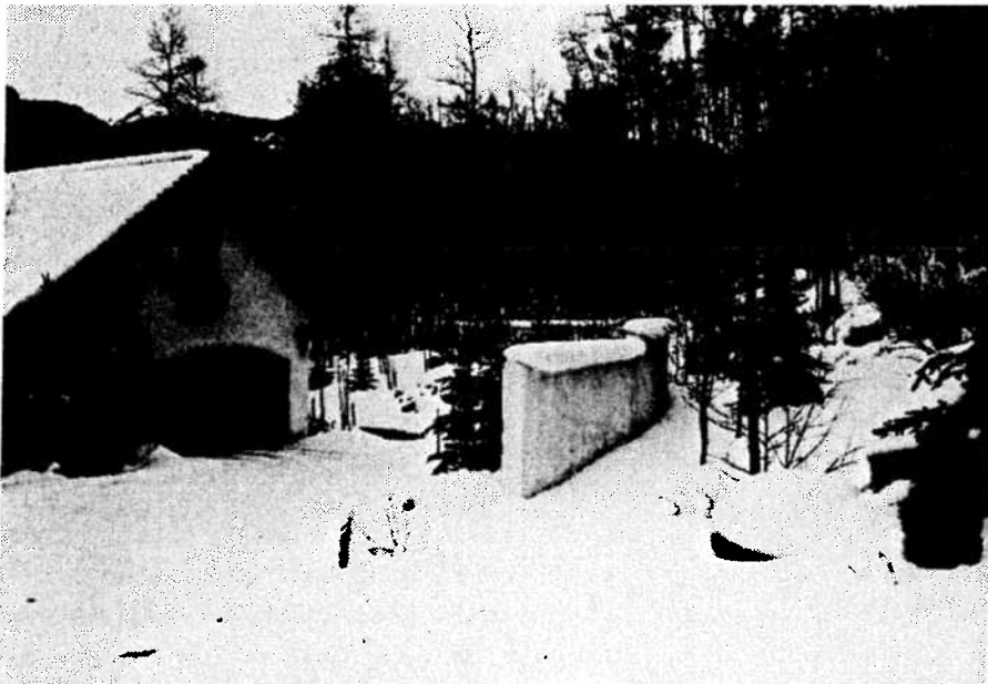
Figure D-7: Floodwall Protecting Residence in Colorado
